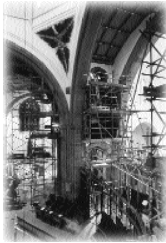
The organ scaffolded during the re-installation
